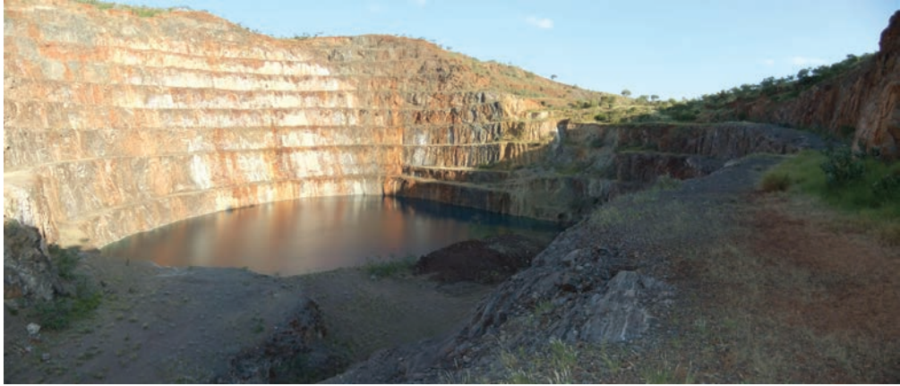
Fig. 19.3. Former open cut mine at the Mary Kathleen uranium project, showing active weathering (i.e. sulfide oxidation) of the side walls and the lack of any rehabilitation of the former pit where water quality remains poor (photo, G. M. Mudd).
