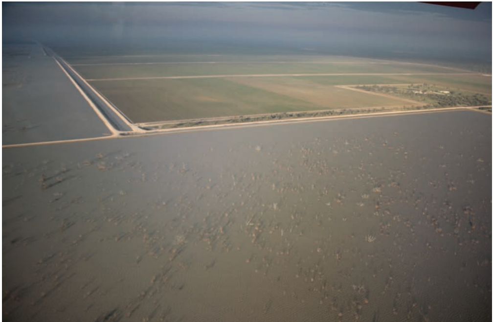
Fig. 14.2. Cubbie Station lies upstream of the Lower Balonne floodplain and has storage capacity to hold more than 500 000 ML of river water in large off-river storages, predominantly to irrigate cotton. This has decreased flooding downstream, incurring significant impacts on downstream communities (photo, R. T. Kingsford).
