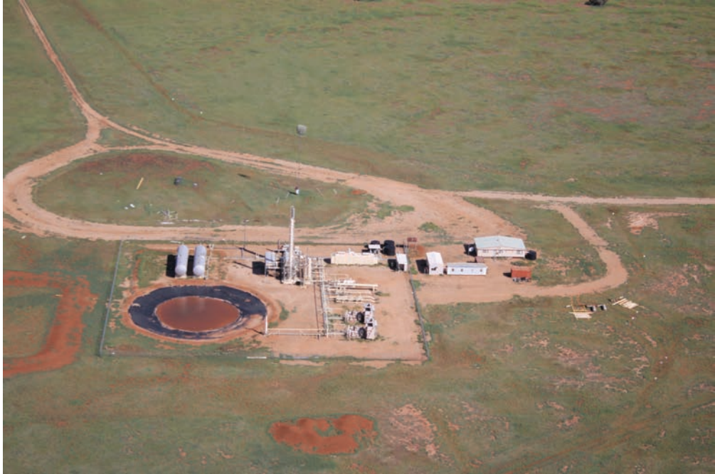
Fig. 19.2. Typical oil and gas production facility in the Cooper–Eromanga Basin of the Lake Eyre Basin, south of Innamincka (photo, R.T. Kingsford).
